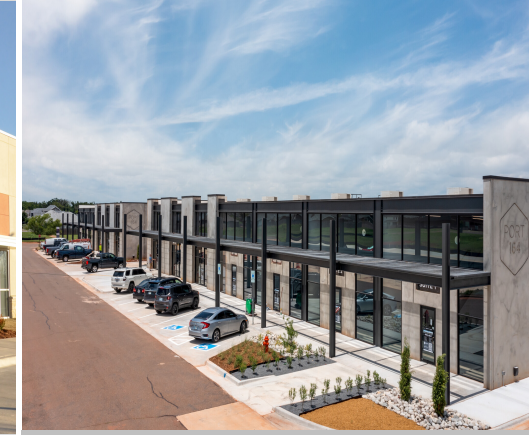
3801 NW 166 th St. Office Park – Edmond, OK
