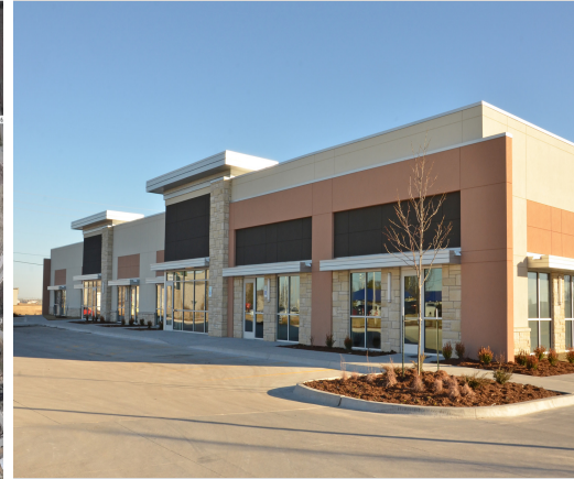
3161 N Webb Rd Office Park - Wichita, KS
